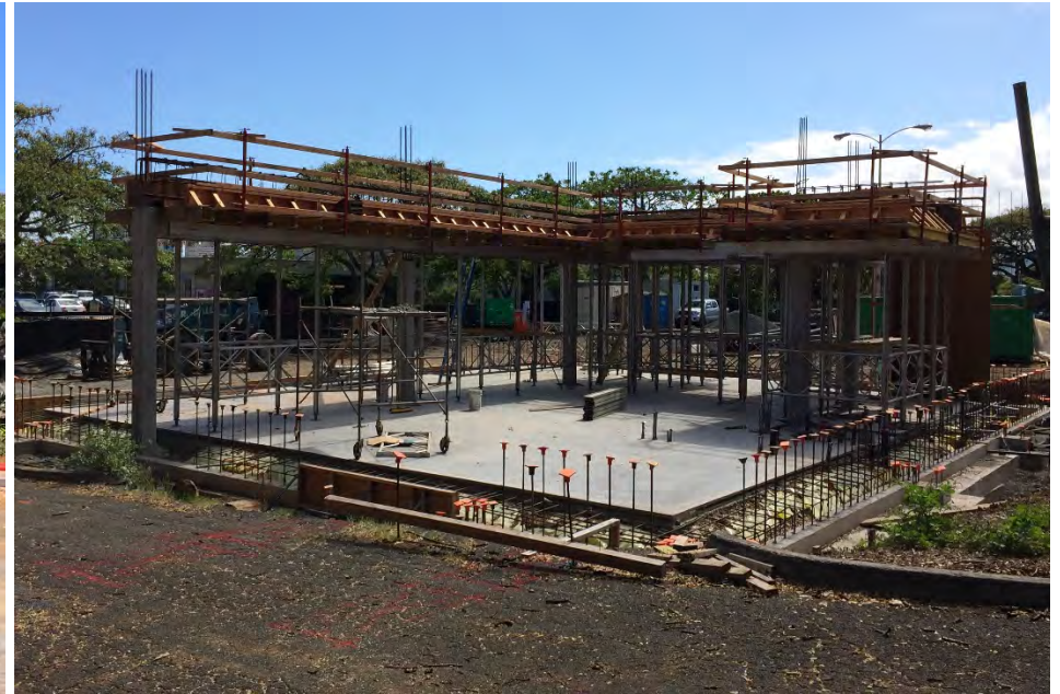
Completed floor slab, interior columns, and forms installed for the beams. Wall precast panels will be installed around the perimeter.
