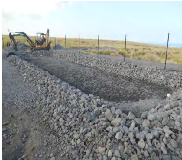
Recirculating Sand Filter
