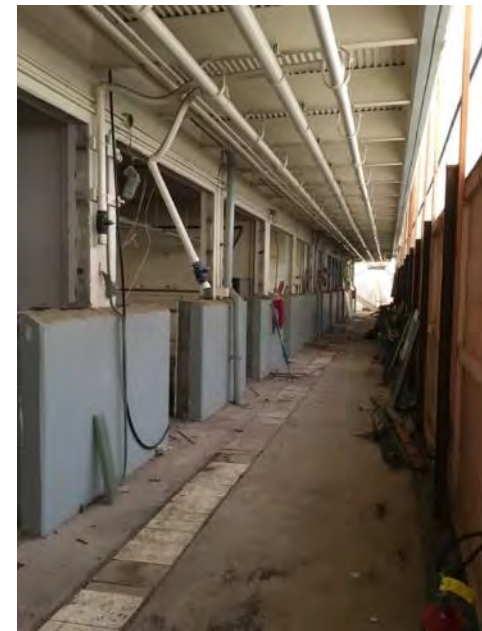
Ground floor exterior walkway of Building 1. At right, construction barricade to separate the work area from the road has been erected. At left, the demolition of the windows and doors is complete
