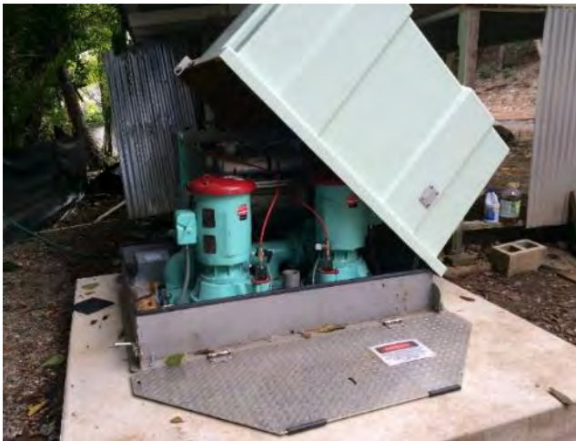
New sewer pump station, which began service on March 1, 2017
