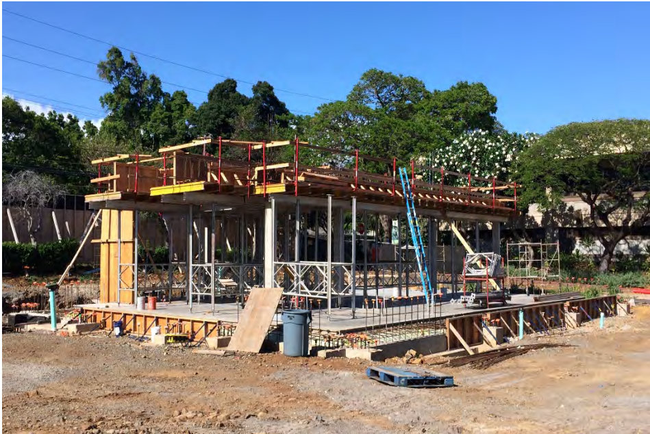
Completed floor slab, interior columns, and forms installed for the beams. Wall precast panels will be installed around the perimeter.
