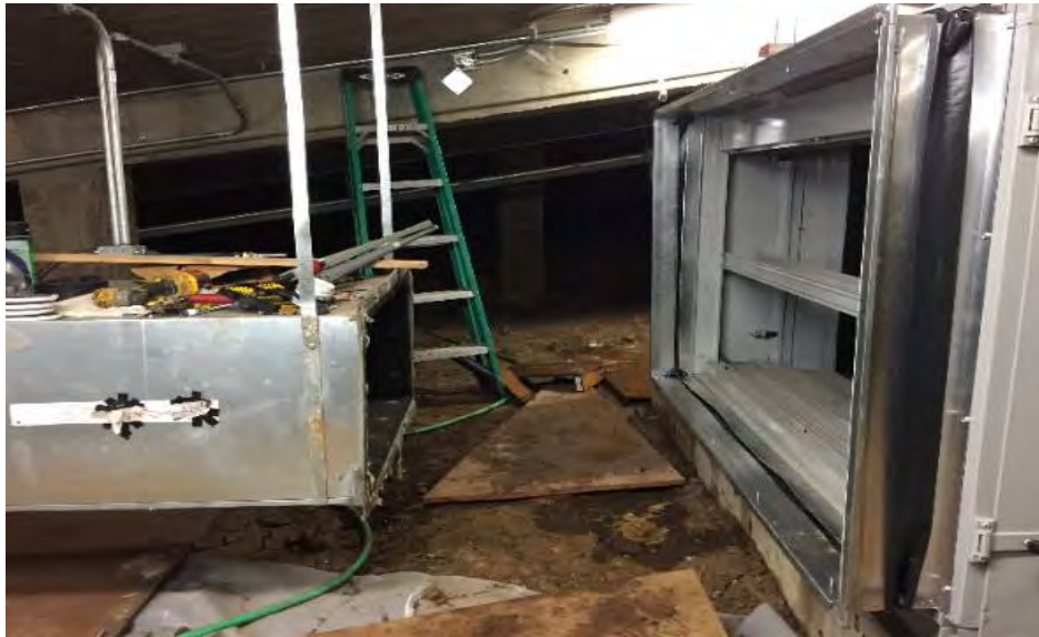
Installation of the new AHU B3 and sheet metal ductwork in the crawl space of Bilger Hall.
