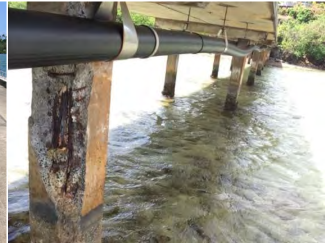
Pile that has deteriorated since the initial investigation and design phase
