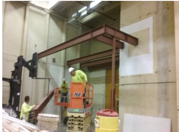
Installation of steel mezzanine
