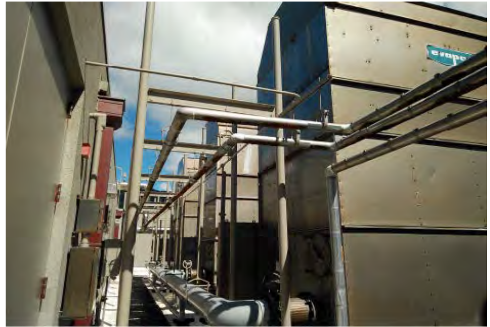
Three existing cooling towers in poor condition will be replaced with two new cooling towers
