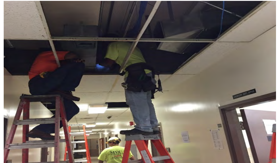
Installation of new sheet metal air conditioning ducts in the 2 nd floor offices of Bilger Hall to provide more even distribution of conditioned air.
