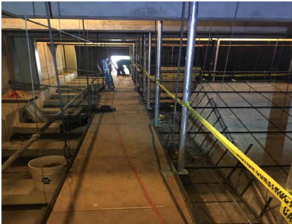
Catwalk above auditorium. Installation of metal rail system
