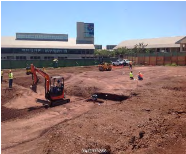
Compaction of soil to prepare for foundations
