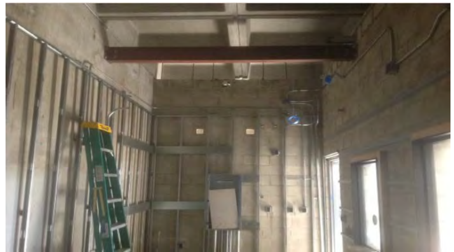
Ticket Office wall and steel framing, utilities rough-in, and windows
