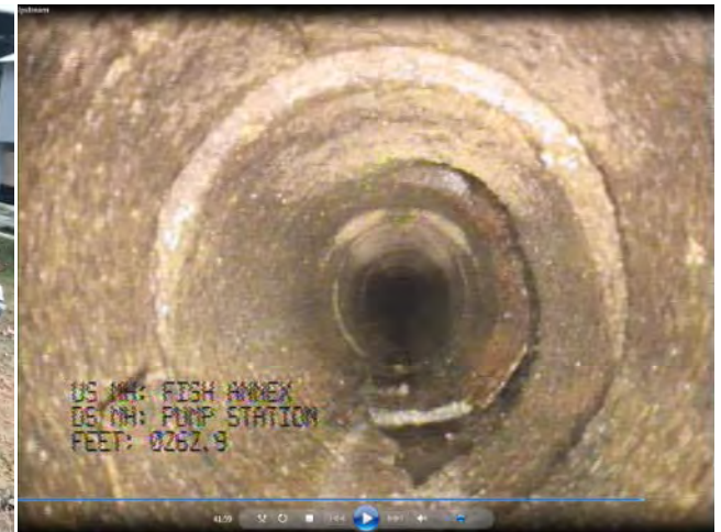
Screen capture of the inside of one of the gravity sewer pipes requiring repair
