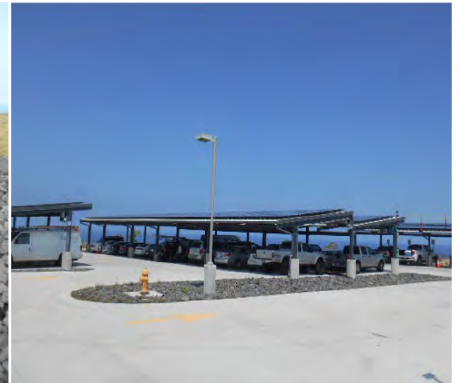
Photovoltaic system installed over parking
