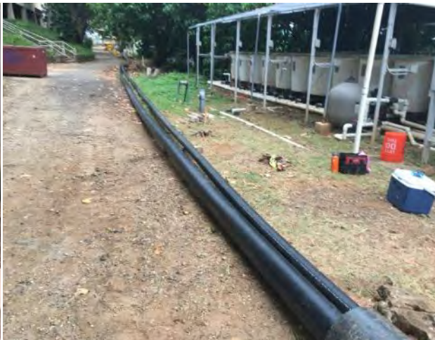
6" sewer line and 4" communication conduit prior to being pulled back from Coconut Island to Oʻahu through the boring
