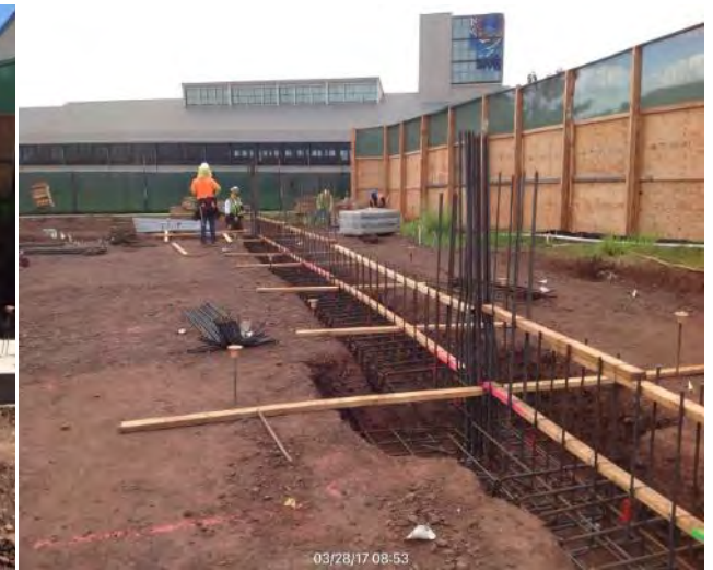
Reinforcing for concrete footings at Administration wing
