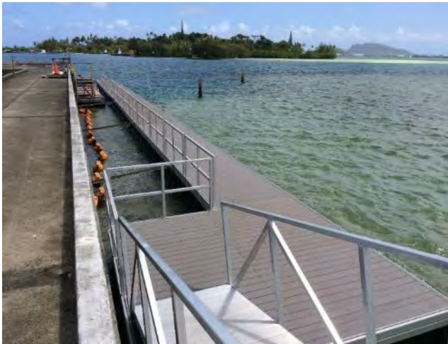
Temporary floating dock has been installed adjacent to the permanent concrete dock
