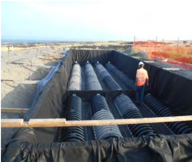
Construction of recirculating sand filter
