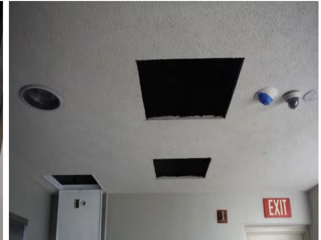
School of Architecture ceiling cutouts for new elevator lobby lights
