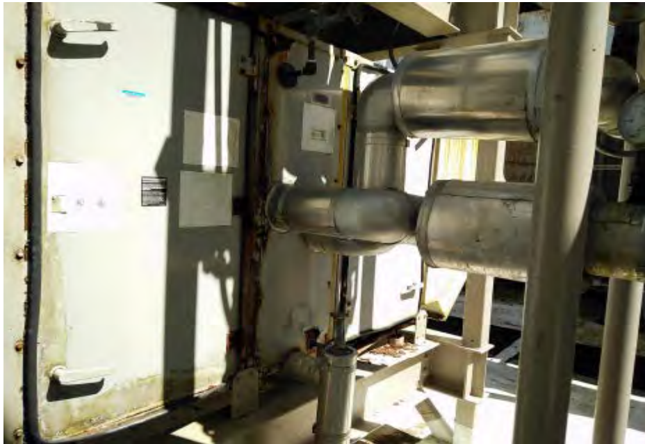
Existing air handlers are in poor condition and badly corroded
