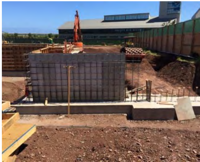
Concrete footings and forms for retaining walls at Administration wing
