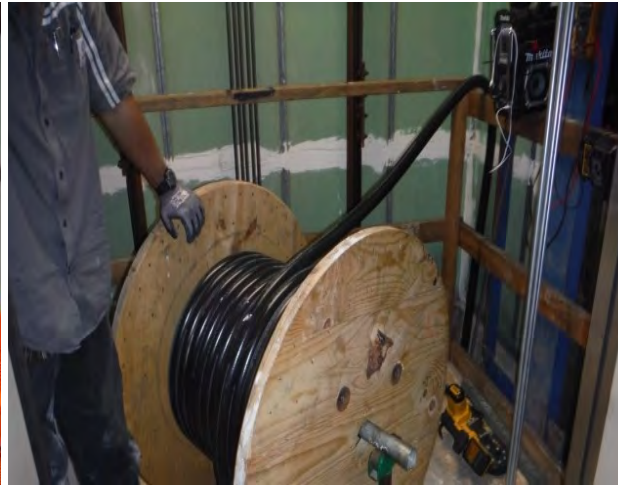
Installation of elevator traveling cable for passenger elevator #2 in POST
